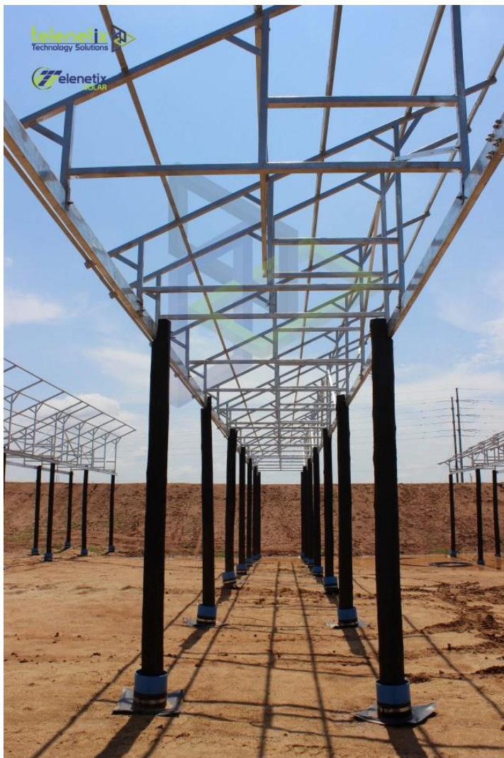
Photograph 1. Penetrating Column connection to the future HDPE lining.
