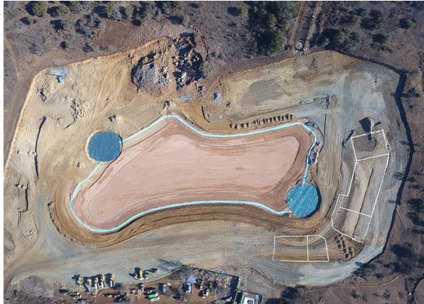
Figure 2: Plan view of the lagoon prior to lining commencement
