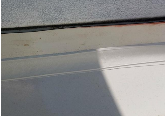
Figure 5: Close-up of the horizontal extrusion weld.
