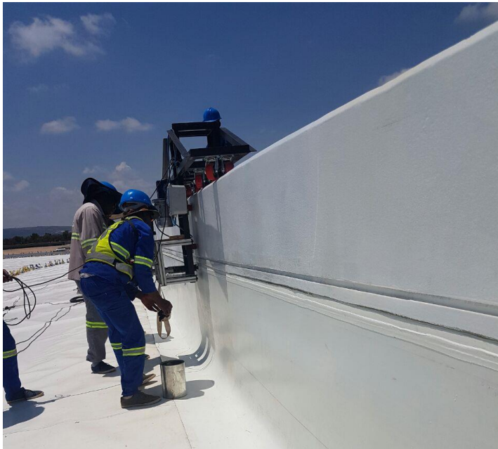
Figure 4: Mechanically-driven extrusion welding mechanism busy with the horizontal extrusion weld.
