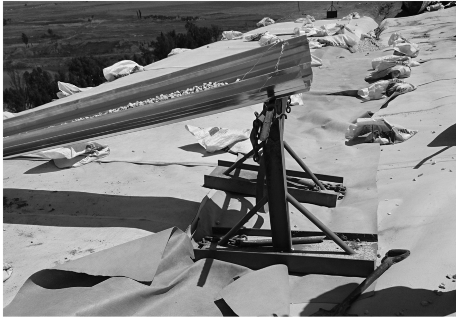
Figure 5. Chute for 19mm drainage stone installation.
