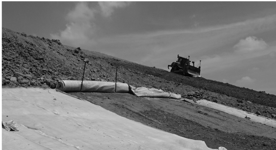
Figure 6. Solution for keeping rolls of geocomposite drain in place on side slopes.
