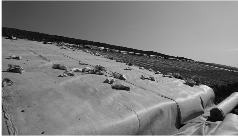
Figure 4. Installation of geocomposite drain in anchor trench.
