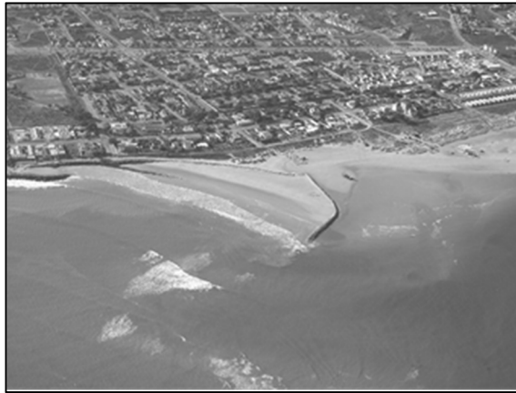
Figure 4: 10 months after the construction of the groyne
