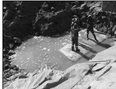
Figure 11: Initial installation of GSC's
