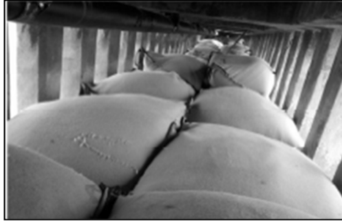
Figure 9: GSC's used to restore the design rip current. (CSCM)
