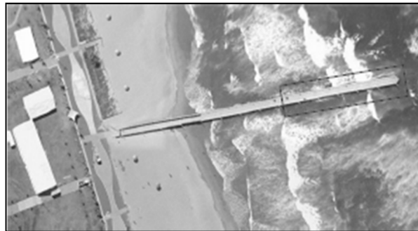
Figure 8: 80m of the seaward deck was removed and replaced by a wider concrete deck (CSCM)
