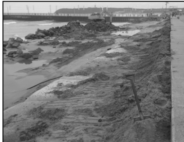
Figure 10: GSC's during installation
