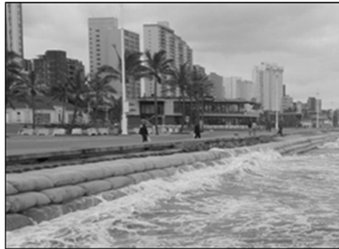
Figure 13: High Sea swells up against the recently installed GSCs
