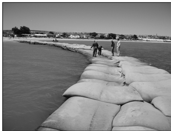
Figure 3: the GSC groyne extending out
