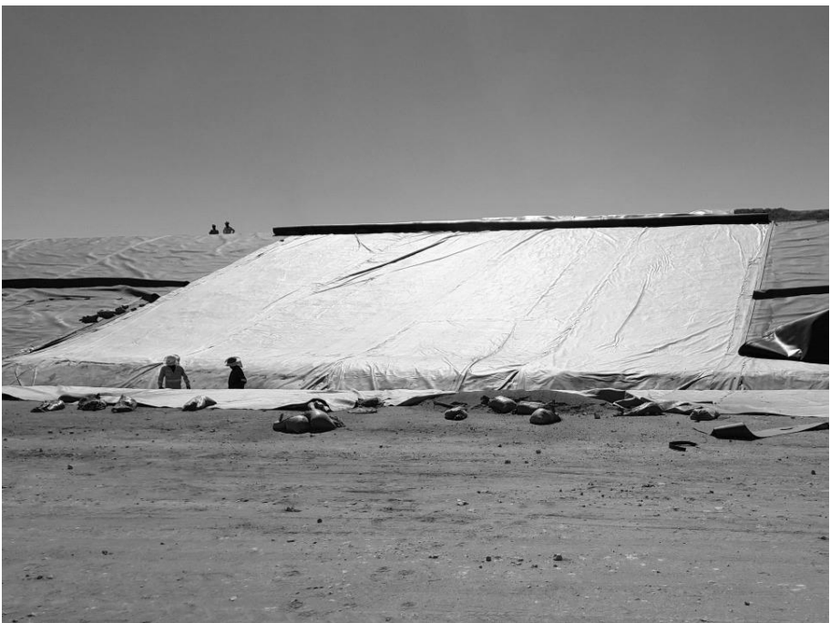
Figure 9. Re-placed geotextile with tacked edges
