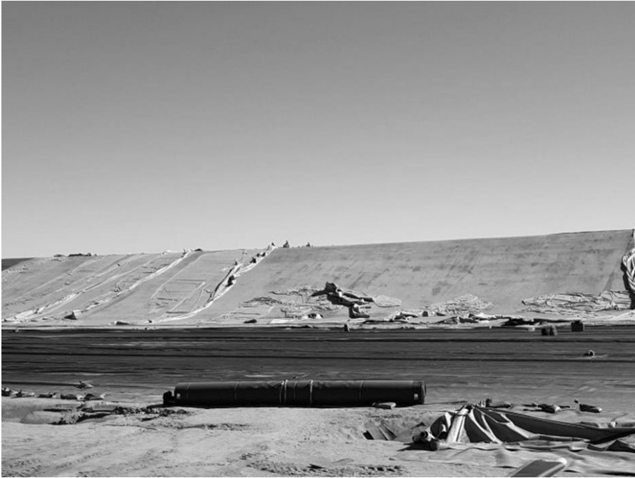
Figure 8. Newly opened (cut) starter wall
