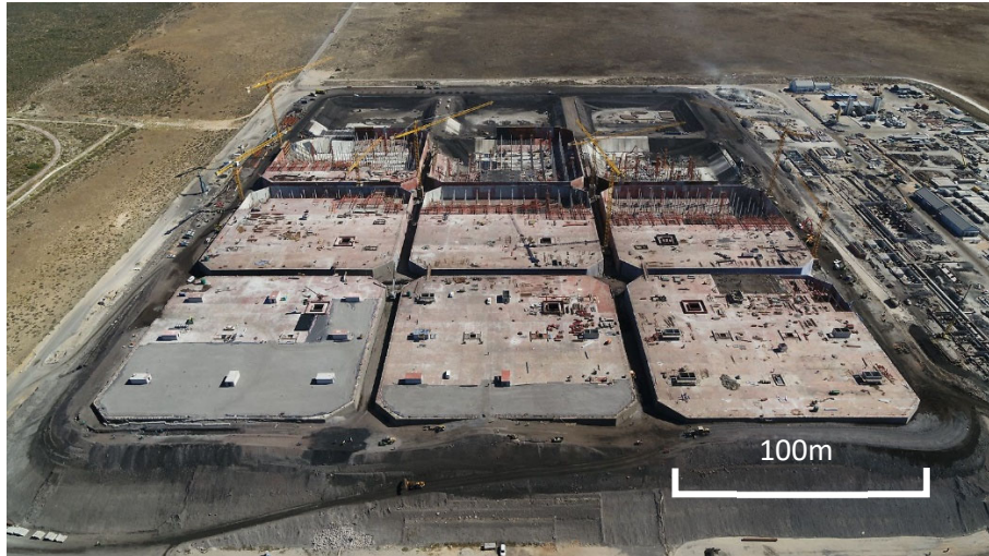
Figure 2: Aerial image of OTMS site during construction. (Image source: www.peri.co.za, November 2018)
