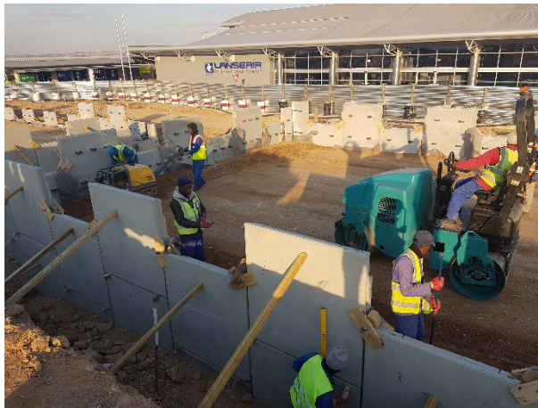
Figure 9. Different compaction techniques used in the backfill
