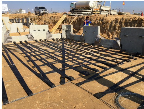
Figure 7: Paraweb reinforcement installed
