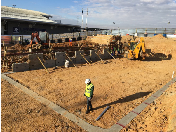
Figure 8. Foundation and levelling pad with first row of panels
