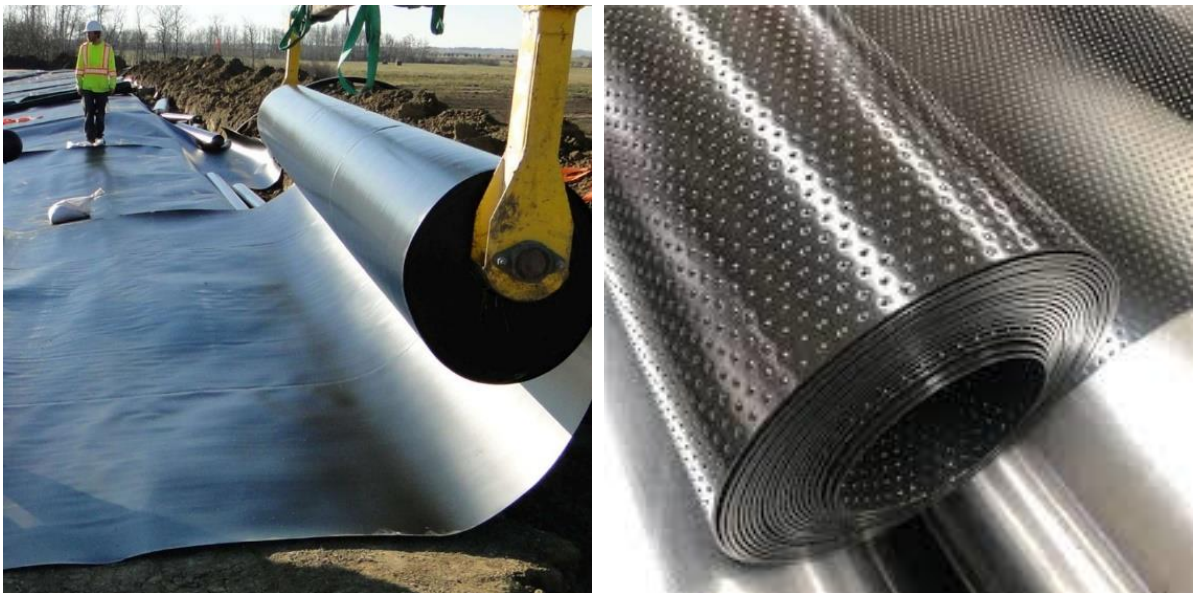
Image: Geomembranes, Smooth (left) and Textured (right)
