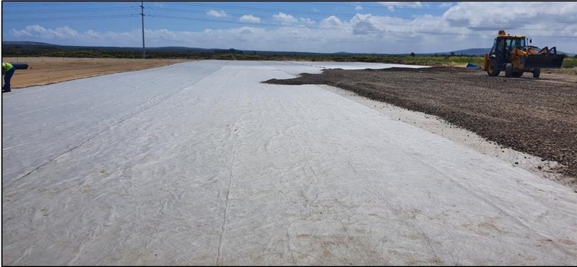
Figure 6. Non-woven polyester geotextile being covered with G5 gravel
