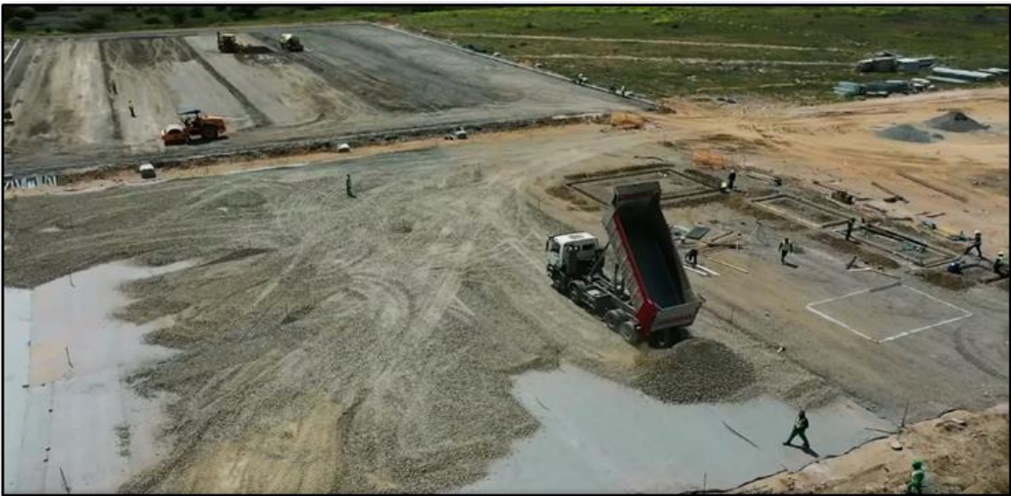
Figure 5. Non-woven polyester geotextile being covered with G5 gravel
