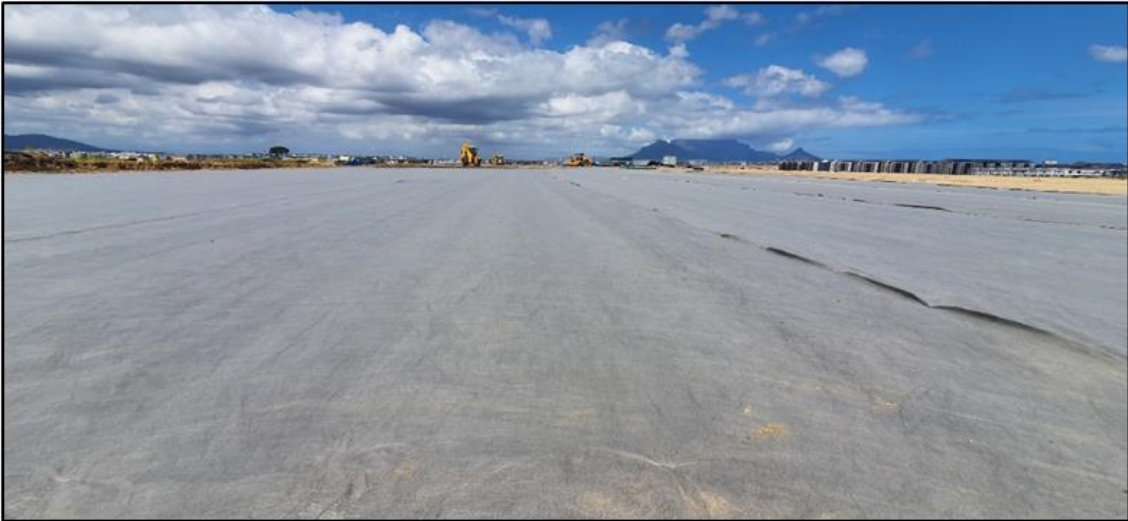
Figure 4. 10 200 m 2 of non-woven polyester geotextile being laid
