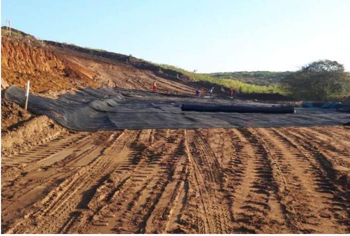
Figure 6: Placing of geogrids with correct orientation
