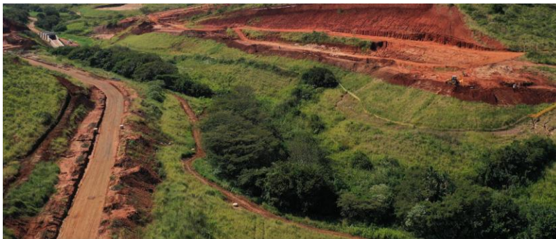
Figure 8: Aerial view of Embankment constructed
