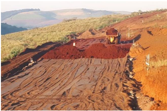
Figure 7: Placing soil to create axisymmetrical condition
