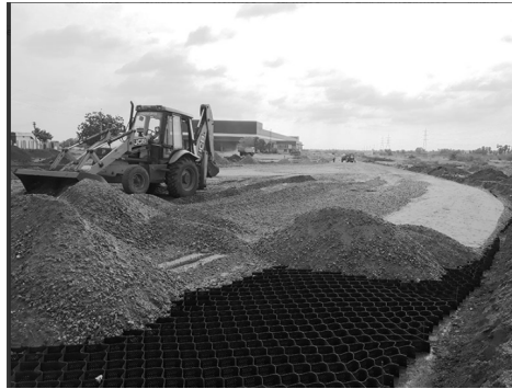
Fig 14. Strataweb® filled with local aggregate
