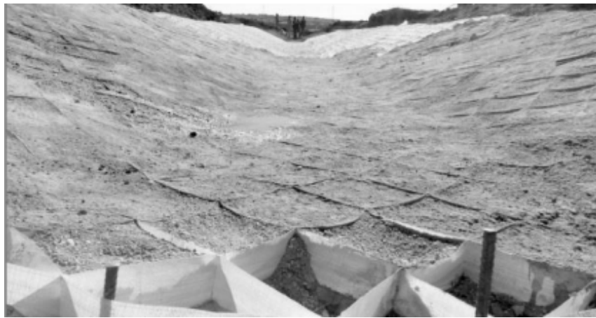
Fig 12. Premix concrete infill
