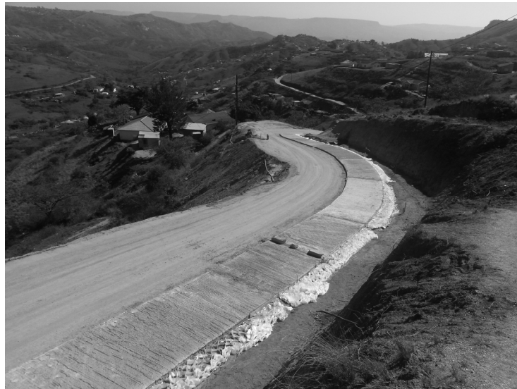
Fig 3. Geocell infilled with concrete for a road
