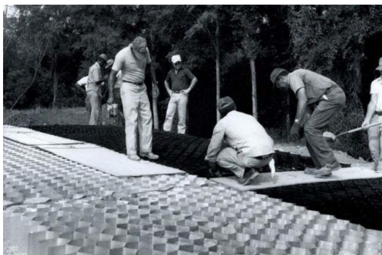
Fig 7. Side by side aluminum and plastic geocells
