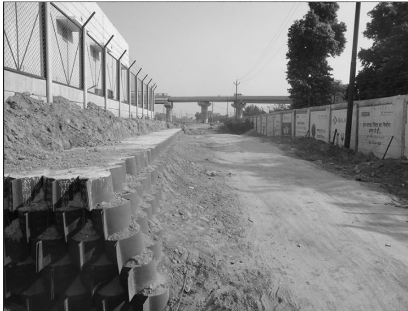
Fig 15. Earth retaining wall using geocells.
