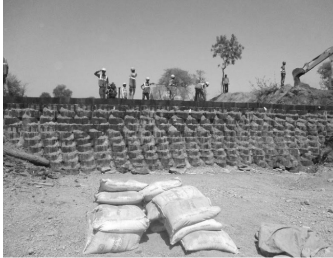
Fig 17. Check dam design
