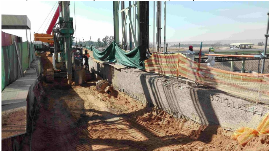
Figure 1-2. Site access below the pipe bridge
